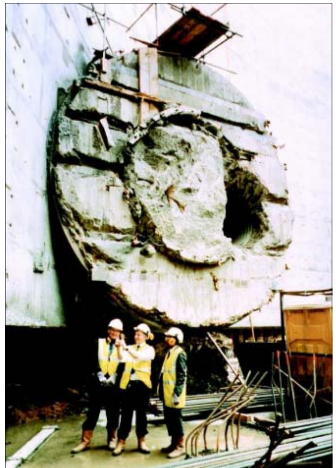
Fig 16 Early tunnel breakthrough
