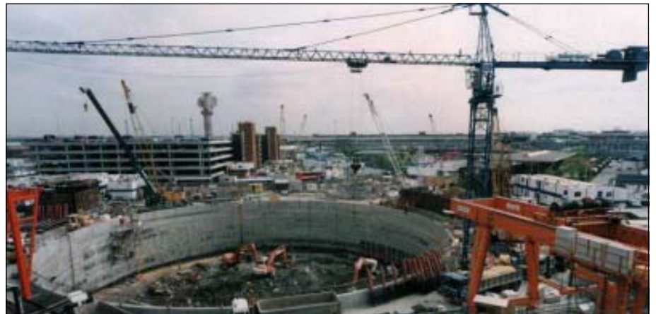
Fig.10 Cofferdam construction, April 1996
