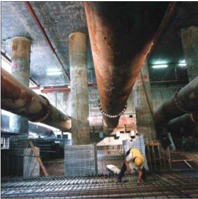
Fig.8 First trial section with 'soft' struts
